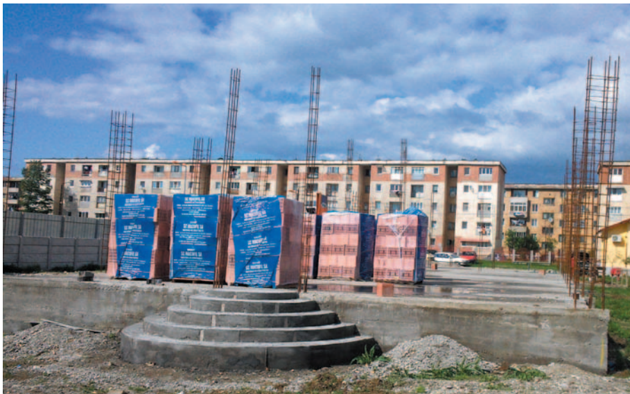
THE CHURCH IN MOTRU UNDER CONSTRUCTION
