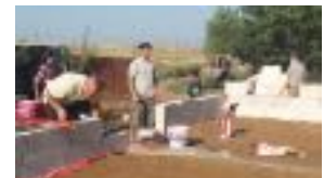
MITICA AND LILIANA FROM CALAFAT NEW HOME BUILD
